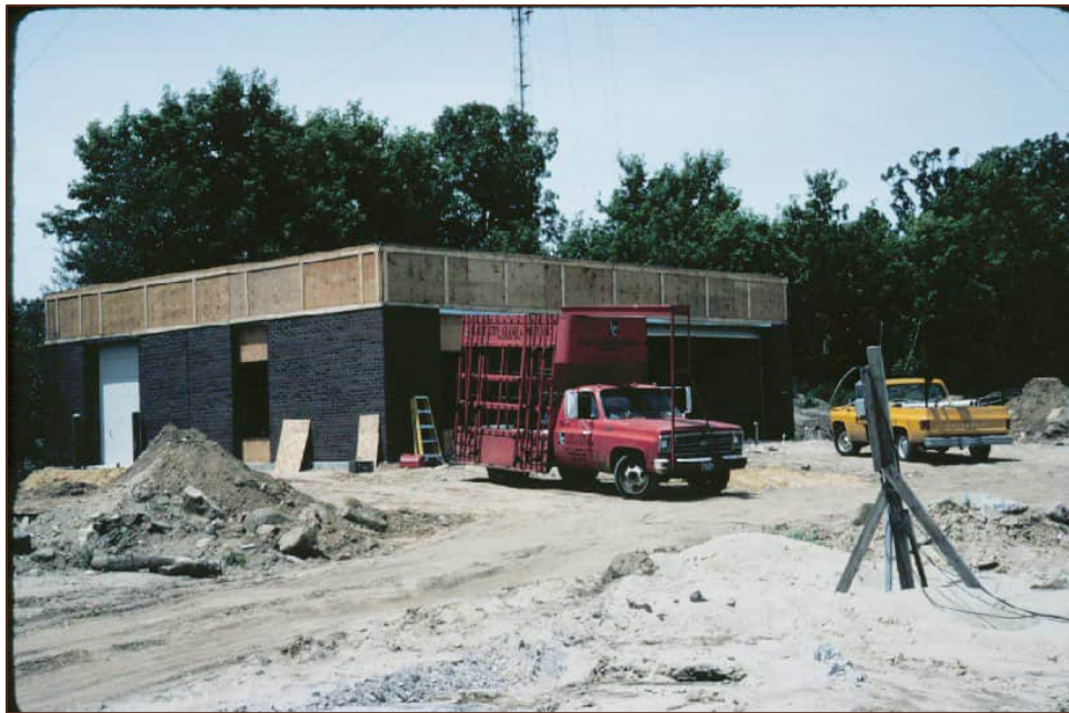
Plate 4. Photograph of NWHC Garage during Construction, ca. 1980 (NWHC Facility Records)
