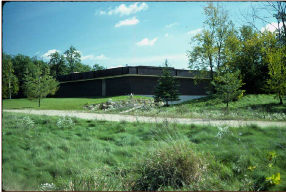
Plate 1. Exterior Photograph of NWHC Main Building Prior to Renovations of Main Entrance (NWHC Facility Records)
